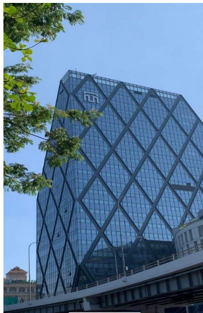
M-Tower (Commercial & Office Building Project_ Chilled Water System)
