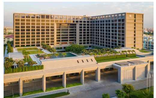
Pullman Hotel Project (Chilled Water System)
